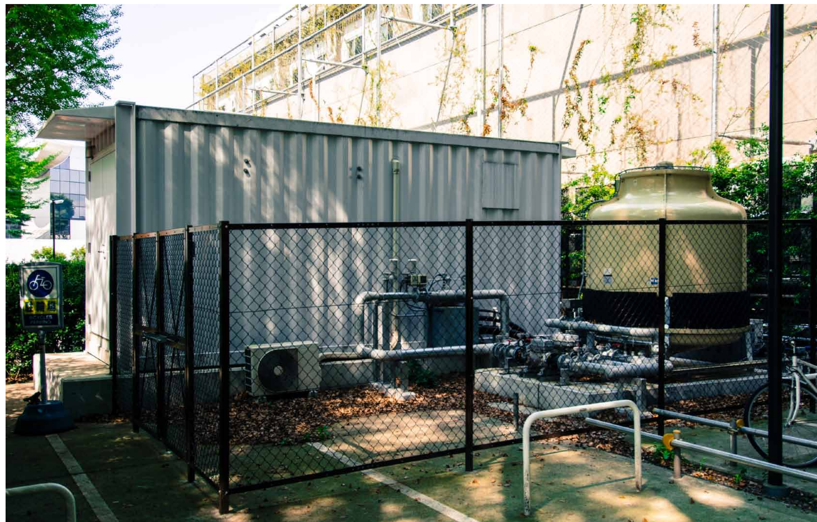
The container-based server room and cooling tower are located beside our computing center building.
