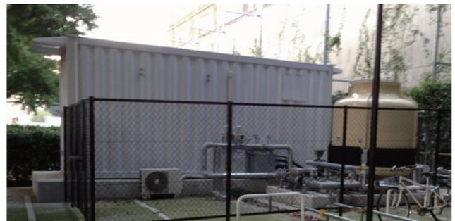
**Fig. 2** Exterior view of TSUBAME-KFC: evaporative cooling tower right next to the 20-feet container for complete lights-out operation and low waterpump power
