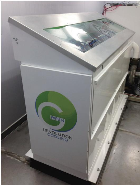
Fig. 3 The GRC Carnot Jet system installed inside the container
