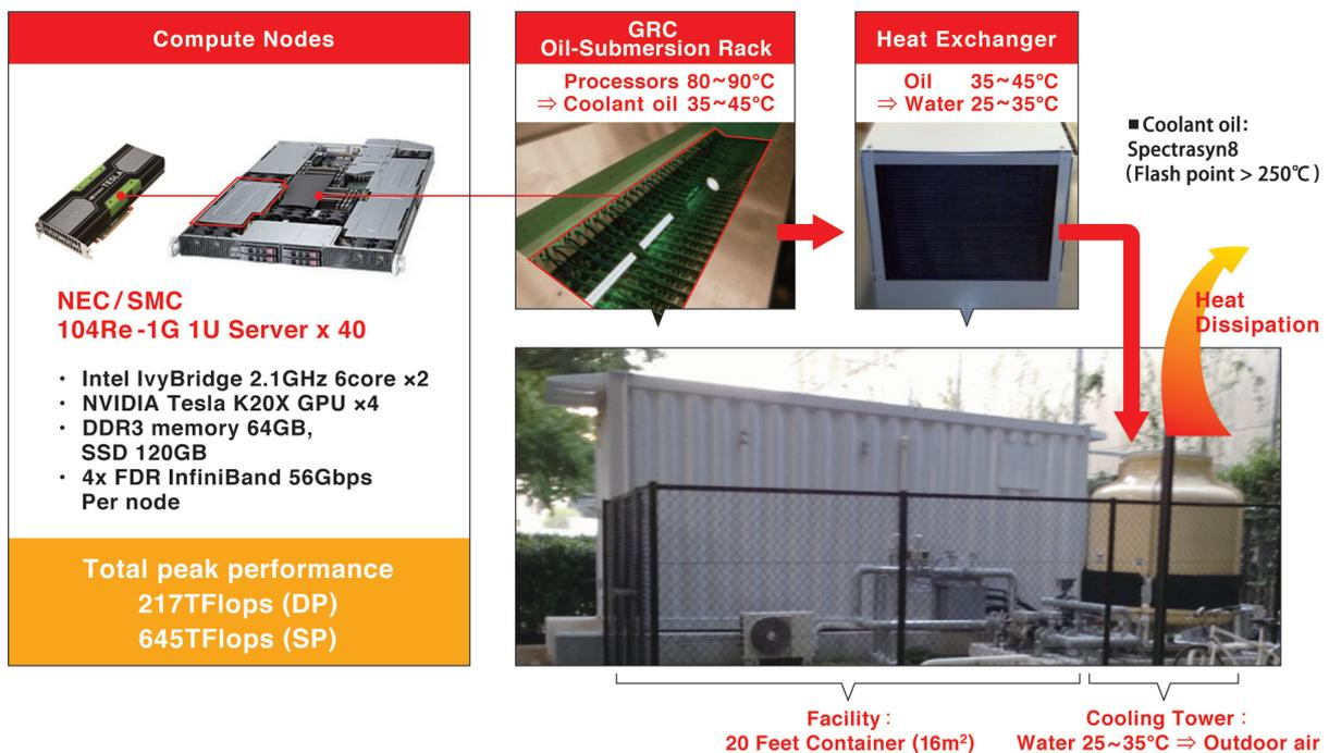
**Fig. 1** TSUBAME-KFC cooling overview: the heat emitted from the server is transferred o submerged oil than to water, than to ambient air.
