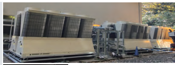
Chilling Units (Cooling Capacity 200 kW/unit)
